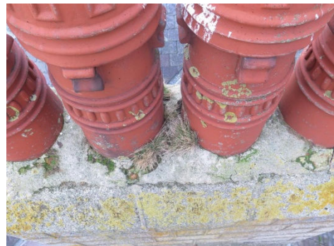
Poor apical tile mortaring and cracked mortar at the chimney haunches, letting in water.
